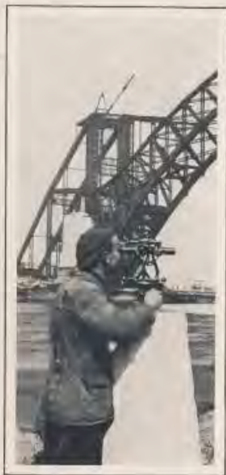
Gurley Precise Transit No. 18-A, mounted on concrete pier, as used at Hell Gate Bridge See page 22 and 23
