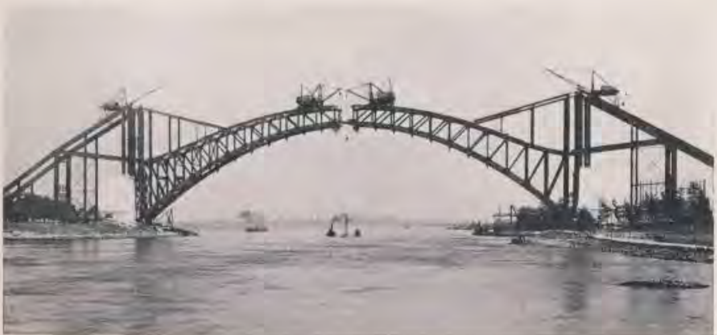
View of Hell Gate Bridge during construction
